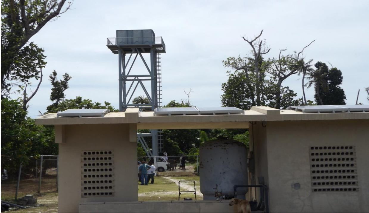
*The new Kayangel State Solar-PV water pumping and supply system, has replaced the electric motor driven pumps of the Kayangel well water systems helping to enable all residents to have water. (photo by S. Abraham(SPREP))*
